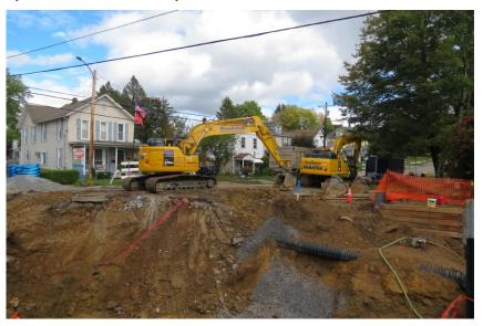
The red line above is where the water line and gas line are to be. The black pipe is a sewer pipe. The worker is about six feet tall and he is directing the shovel driverto dig where red line was..
