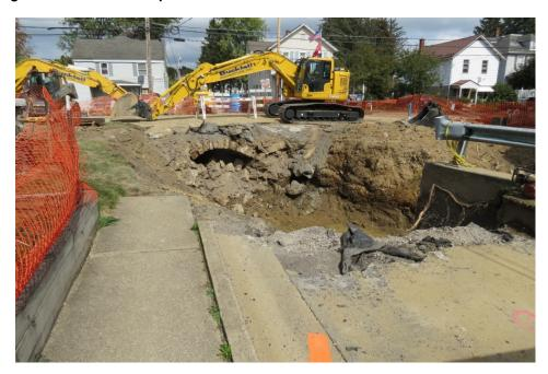
The next picture shows the stones that make the arched roof of the bridge a little more to see how it has to be removed. Now I didn't measure the stones, but my rough guess is that they are about three feet long by 18 inches wide and a foot thick. It starts under the house behind the 2 power shovels.
