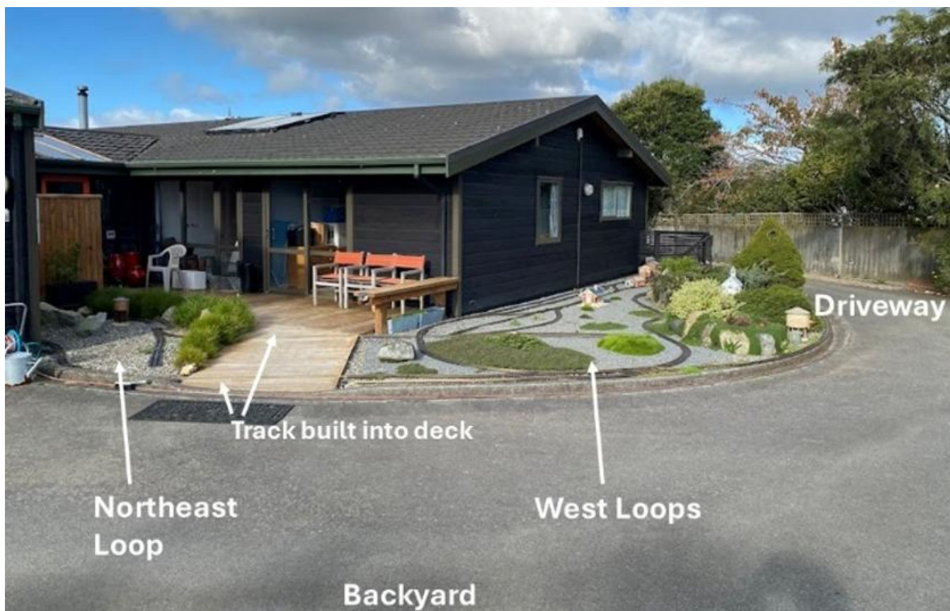
Location of the Northeast Loop and West Loops sections connected by track crossing the wooden deck (looking south).
