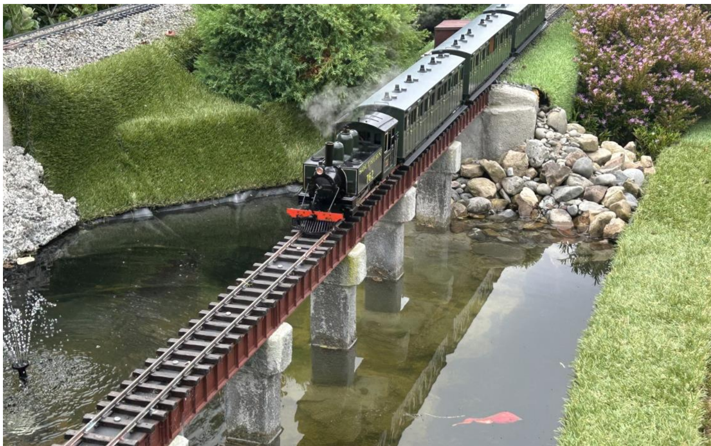
Derek's Accucraft Lyn on the pond built beam girder bridge. Getting the right angle for the best reflections in the pond is still a work in progress.
