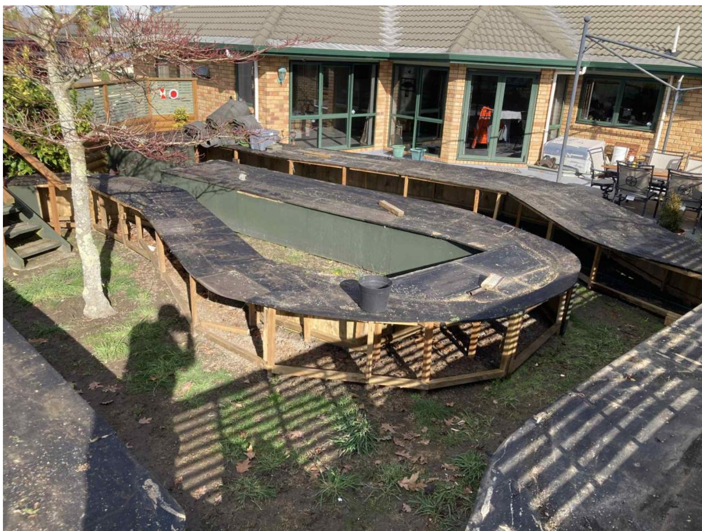
Stripping the old layout of scenery, artificial grass and side cladding.
