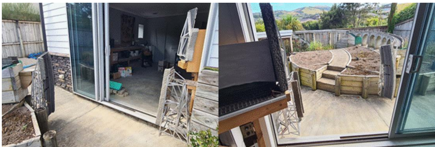
Views of the folded away edge boards from outside and inside. The hinged supporting legs tuck up between the main frames and adjoining support structures when stowed as depicted here.
