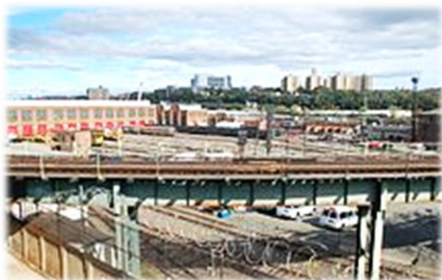
207th Street Yard from the southwest – note the Museum cars.
