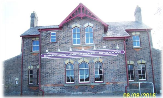
The station with identifying sign.
