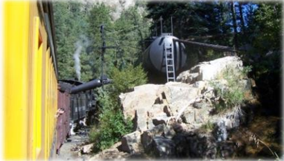
A spring fed tank car body serves as an unusual water tank on route. When the tank is full the excess runs back into the spring.
