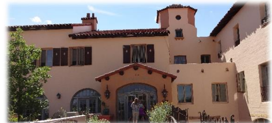
We stopped for lunch at La Posada, the restored Harvey House hotel and restaurant alongside the (now) BNSF tracks. The food was good, the hotel interesting and the long BNSF freights a joy to watch.
