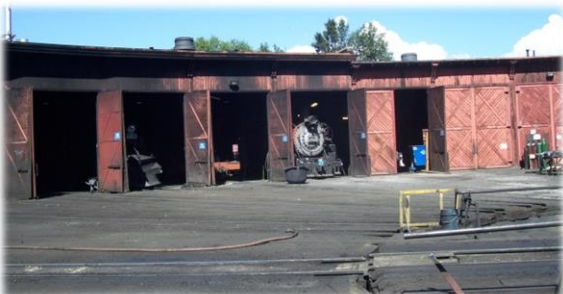
A partial view of the D&SNG roundhouse. The turntable is pneumatically powered, but so well balanced that it can be turned by hand.
