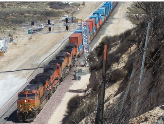
BNSF double stack train enters Cajon Pass. Those wavy lines to the left are rail for the third track that is being added.
