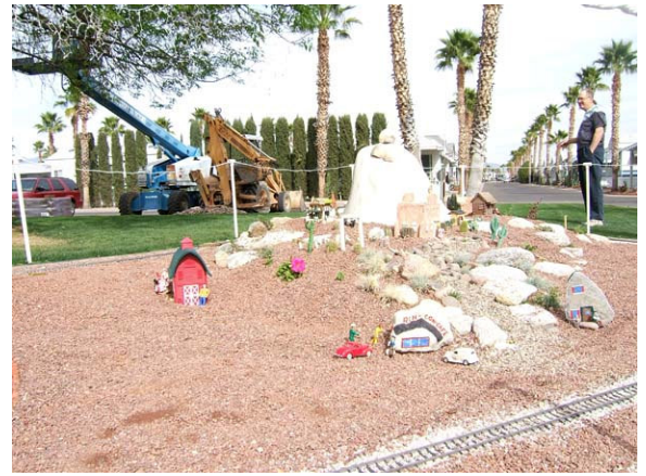
Heavy Equipment parked on the site of the future expansion of the Rincon RV Park Railway
