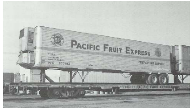
One of the refrigerated truck trailers that made refrigerator cars obsolete.
