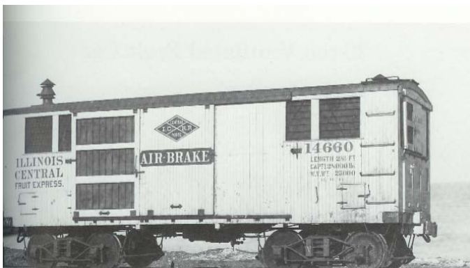
Early Ventiladed Box Car used to ship fruit
