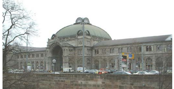
The main Nurnberg Railroad Station (cloudy day).
