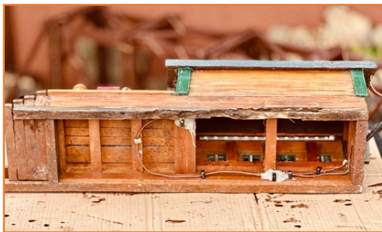
Rat damage at the foundation of the Mine Station.
