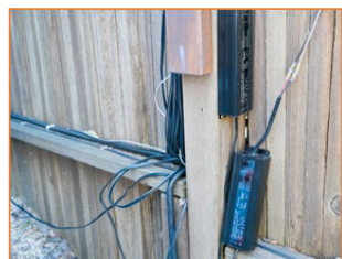
New 12-volt transformers for lights and sounds.
