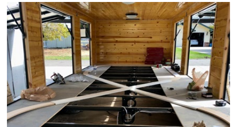
Early stage of figure 8 track layout laid over window-level raised floor.
