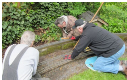
Assisting with track repairs.
