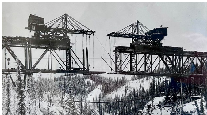
In 1910, crews worked from both sides of a 238 foot deep gorge to complete the Kuskulana River Bridge to transport copper from the Kennecott Mines.
