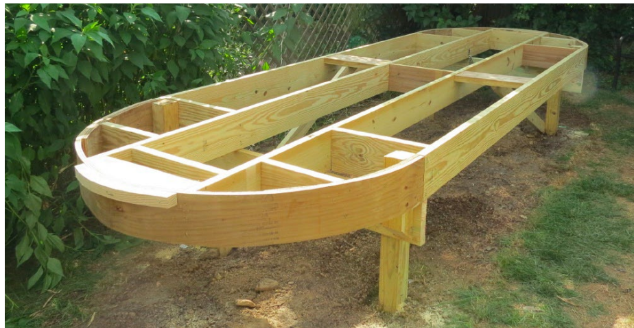
Base structure completed with spacers and supports all in place.
