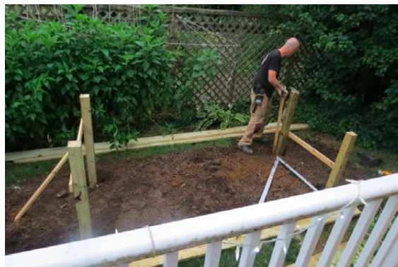
Making sure posts are level and upright.
