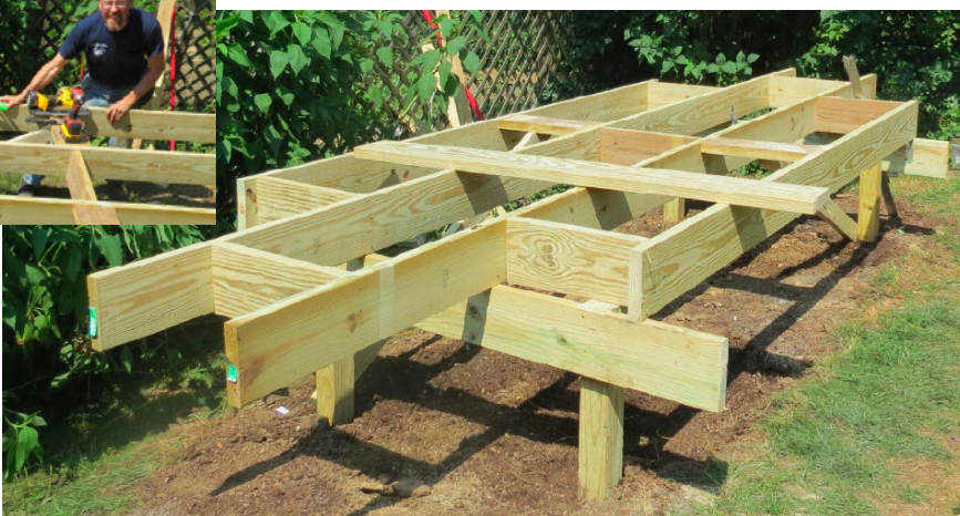
Base structure for table layout with spacers added for strength.
