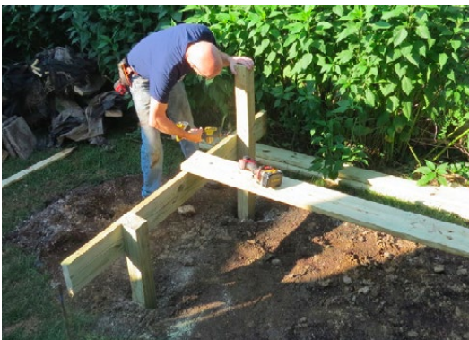
Attaching end board to post.
