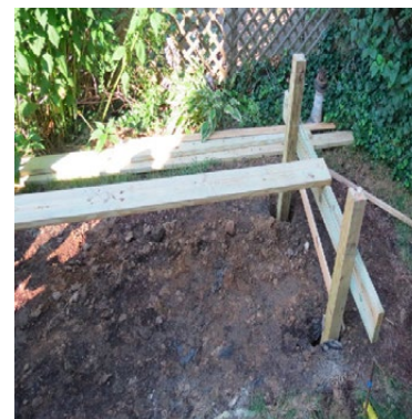
End board & temporary middle spacer in place.
