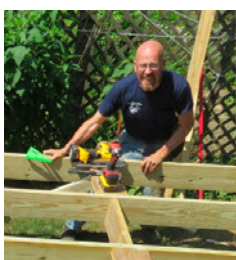
Attaching end board to post.
