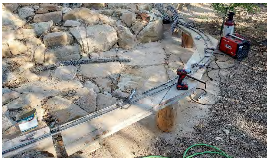
Photo 4 Welding in the viaduct crossmembers.
