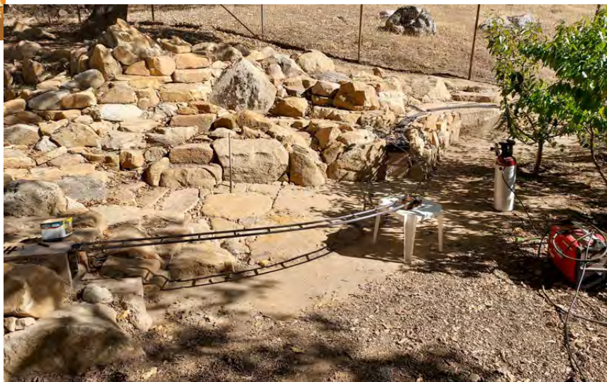
Photo 10 Viaduct top rail before welding on flat stock. A-frame tower supports will be placed between the rail to complete viaduct.
