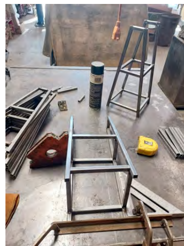
Photo 7 Connecting A-frames together to create towers.
