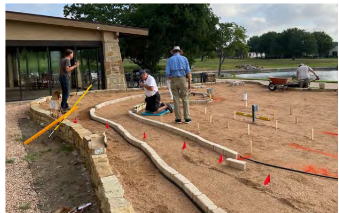
Lower track base stones set in place following hose layout.
