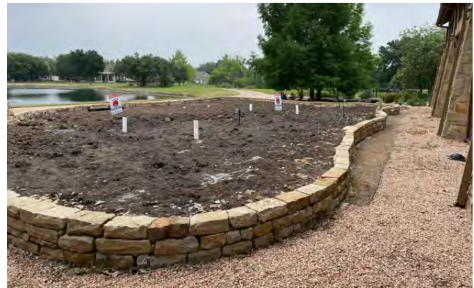
Raised bed retaining wall and dirt bed with drainage.
