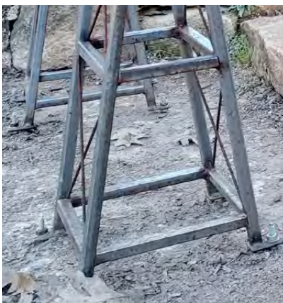
Photo 12 a & b Leveling the rail using Wej-it bolts, nuts and washers at the tower base after reattaching tower to crossmembers.
