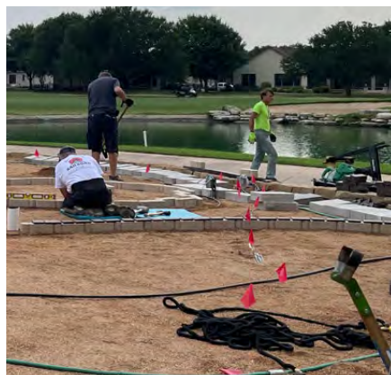
Working on the base for the lower track.
