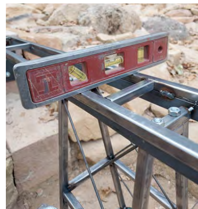
Photo 12 a & b Leveling the rail using Wej-it bolts, nuts and washers at the tower base after reattaching tower to crossmembers.
