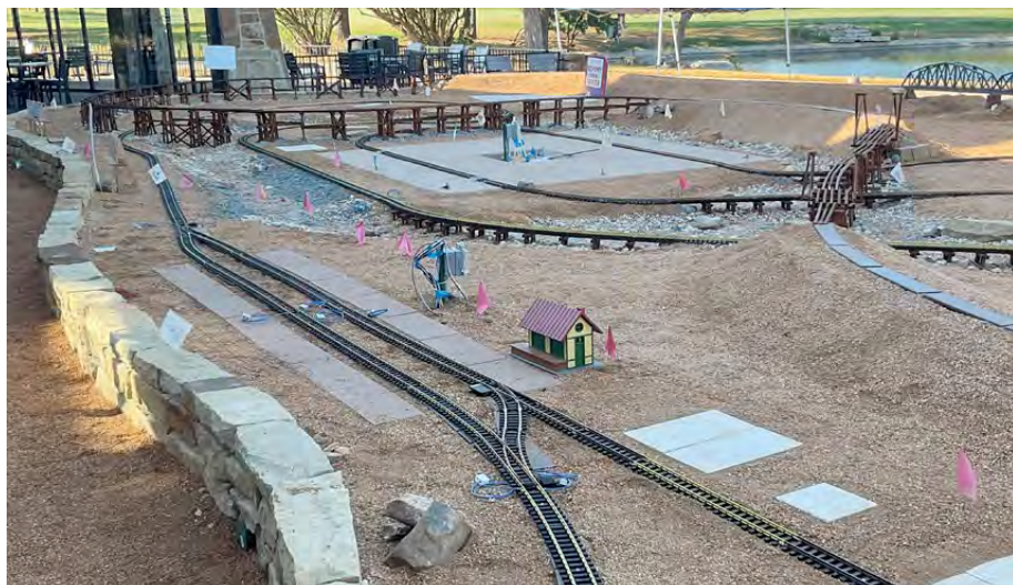
Engine shed & building foundations, including town square.
