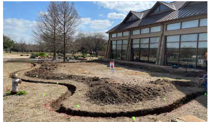
Raised bed footings.
