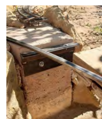
Photo 3 End plate attached with Wej-its supports a rail for the viaduct.
