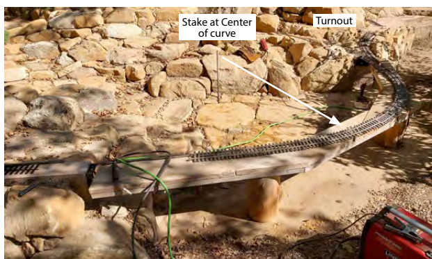
Photo 2 Laying out the curve on a temporary bench.
