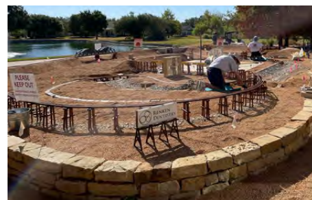
Upper track trestles being assembled.
