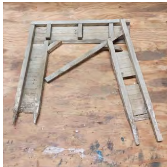
Photo 1 The old timber portal, looking worse for wear.
