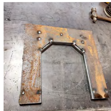
Photo 8 Welding the backing plate on.
