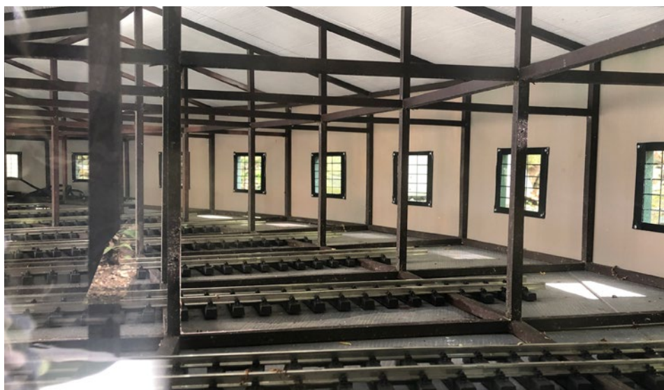
The PVC framing and walls are painted before the roof is attached. The light tan walls will reflect light on the locomotives inside.
