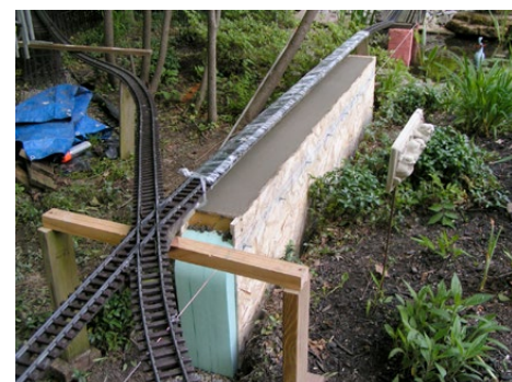
Fig. 6: The first section, poured
