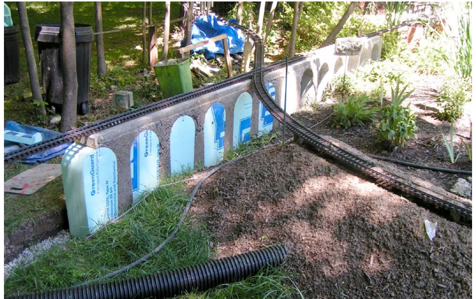
Fig. 8: First two sections poured
