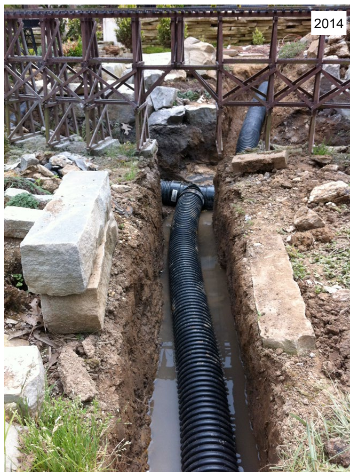
French drain pipe before packing in gravel "roadbed."
