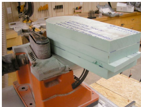
Fig. 3: Smoothing the arch
