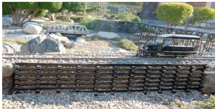
The stacked acrylic cribbing is held together with threaded rods & nuts and stabilized with fill dirt & grit.
