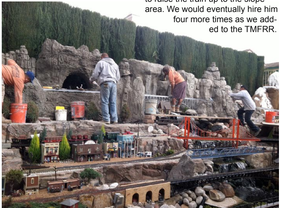
Building up the concrete Utah-look Red Rock Canyon and mountains.
